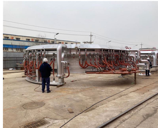
Finished Upper Shells
